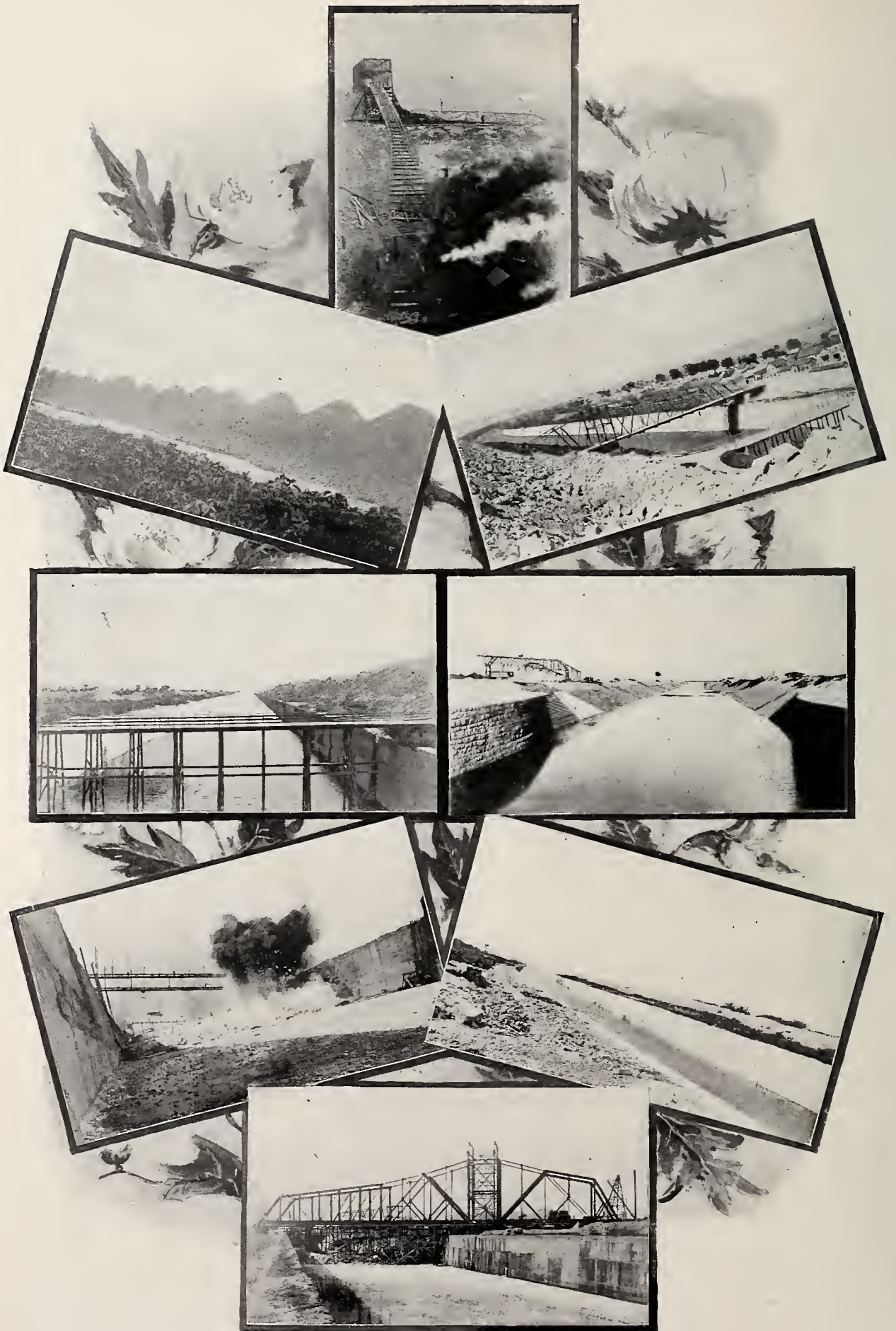
VIEWS OF DRAINAGE CANAL.
